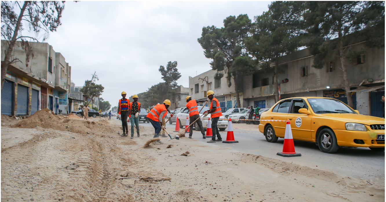
TRIPOLI (LIBYA). Clearing of debris and unexploded devices in municipality of Abu Salim, Greater Tripoli. Photo: ©UNDP Libya
